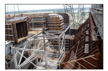
SEI teamed with Sargent and Lundy on Ameren's Coffeen Unit 2 precipitator project. This was a \$12 million engineer, fabricate and supply project for the ESP and associated ductwork. SEI designed and executed a Physical Flow Model of the ductwork from the air pre-heater to the ESP inlet . SEI also designed the duct supports, access walkways and foundations. This project included 611 tons of ductwork and 275 tons of structural steel.
