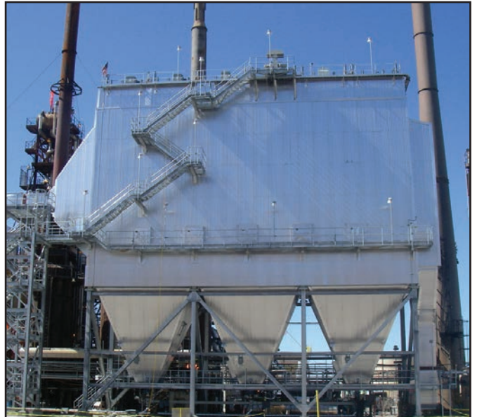
15,000 Barrels Per Day FCCU - ESP
