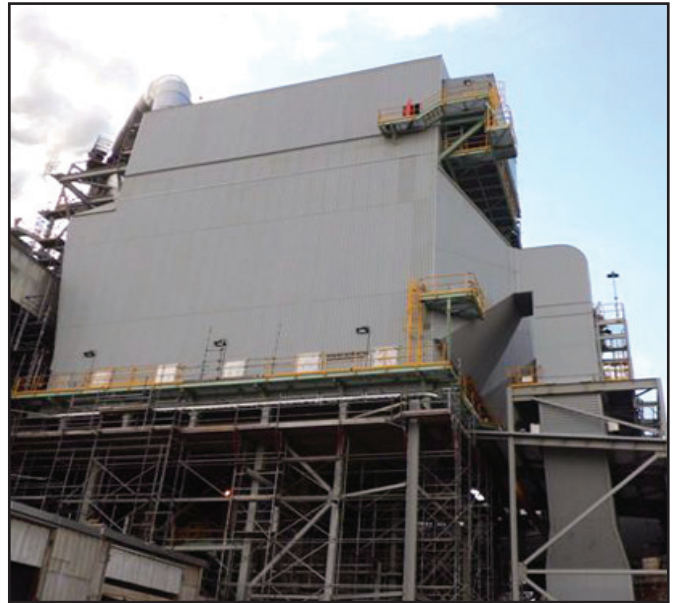
3.75 MM LB/Day of Solids - Recovery Boiler
